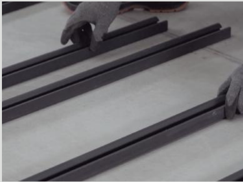
1 REPLANTEO DE RASTRELES. PLANNING THE LAYOUT OF THE BATTENS. IMPLANTATION DES TRAVERSES. УСТАНОВКА ЛАГ.
